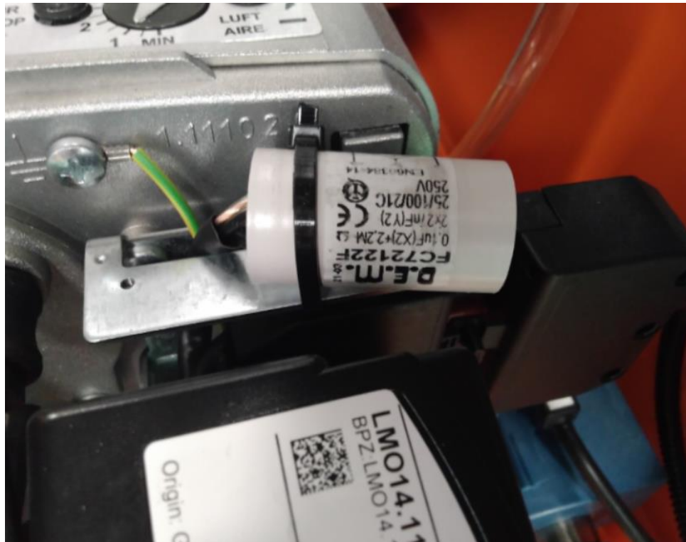
Burning unit radio interference filter
