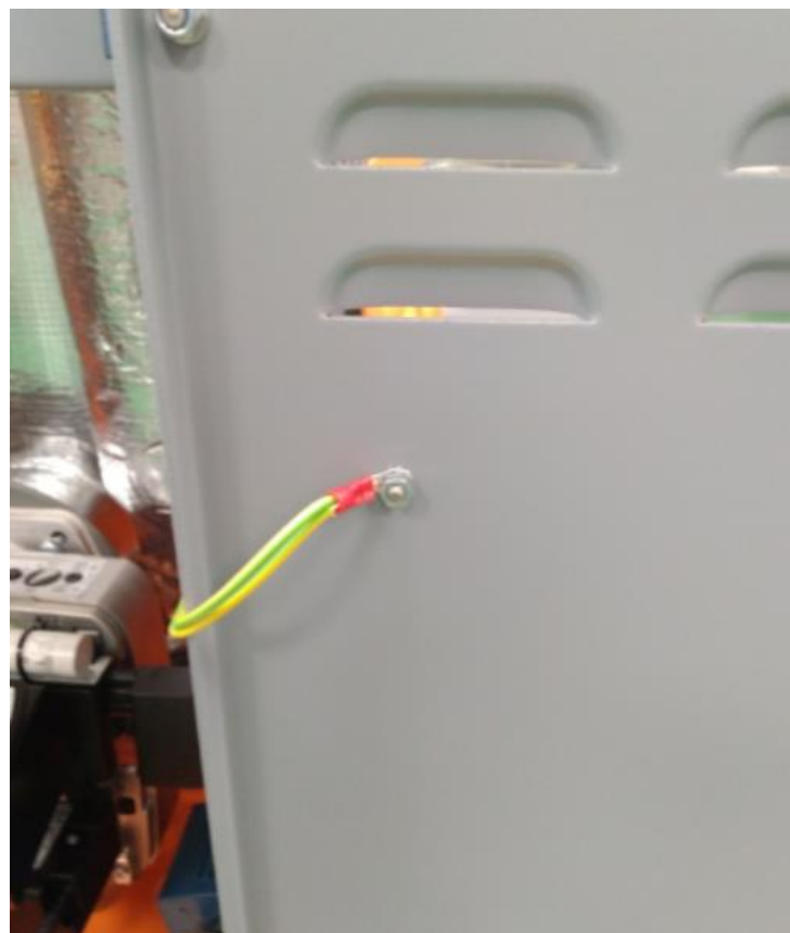
Earthing connection on hinged door
